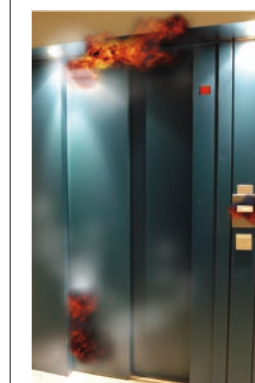
Fire-testing of lift landing doors is only done by applying EN81-58
